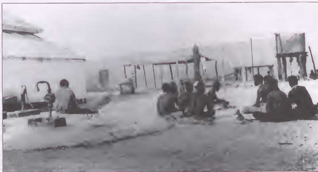
Fig. 3. Photograph of subterranean tank in Area A, looking toward eastern perimeter fence. Note concrete lid, pumps, drainage channel and washstand and tub (in background). Photograph of unknown date but almost certainly within the period 1910-1930s. (Photo: Museum and Art Gallery of the Northern Territory).
